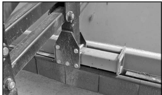
Figure 40. Strut Uprights Installed
